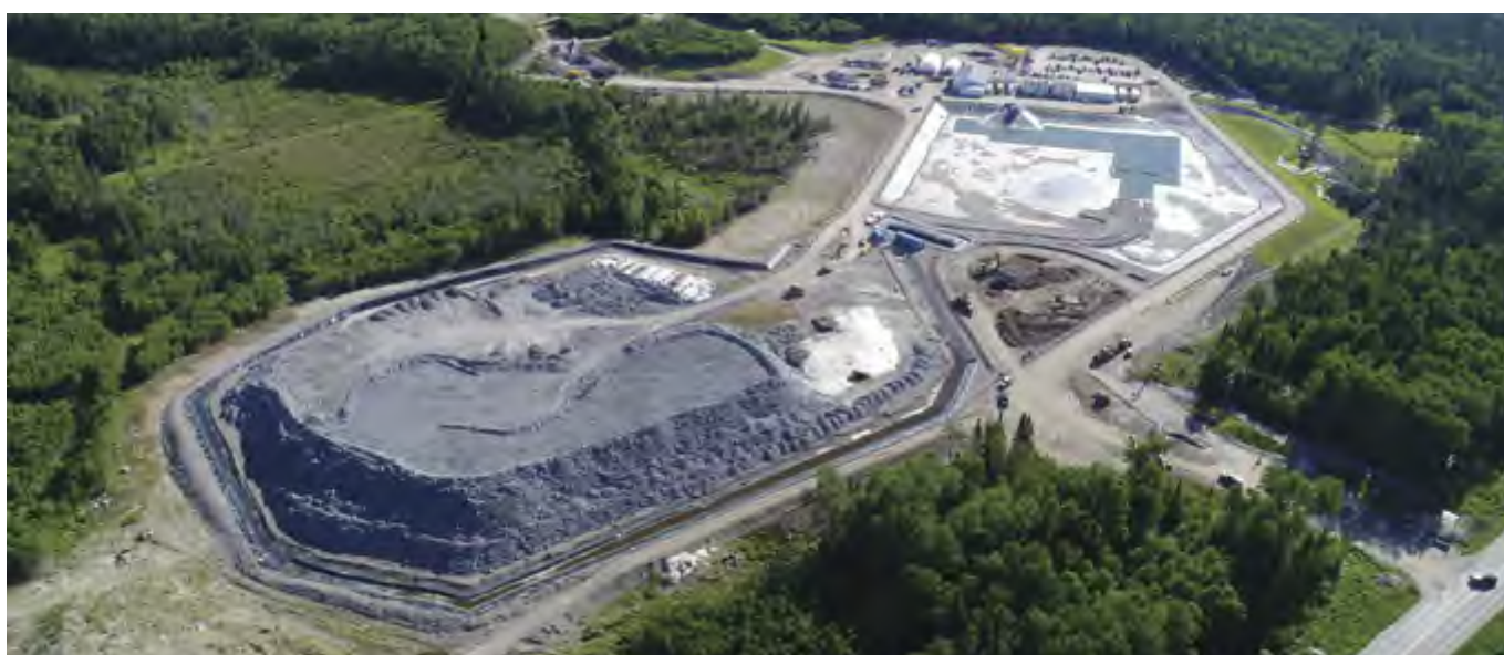
Newmont Goldcorp's Borden mine has been designed to integrate a range of energy efficiency technologies, including ventilation on demand, electric underground equipment, the elimination of compressed air networks and a switch to compressed natural gas instead of propane for heating.
