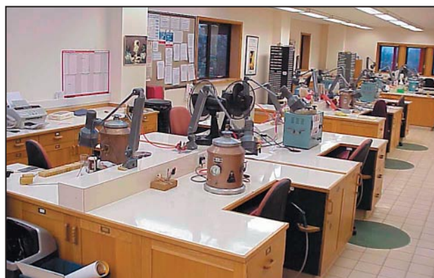
Figure 11 - Group of 4 work stations. Services are routed from the floor up into the centre of the group
