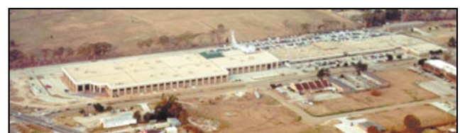
Figure 2 - Aerial photograph of the global headquarters of Stuller, Inc. during expansion to 600,000 square feet
